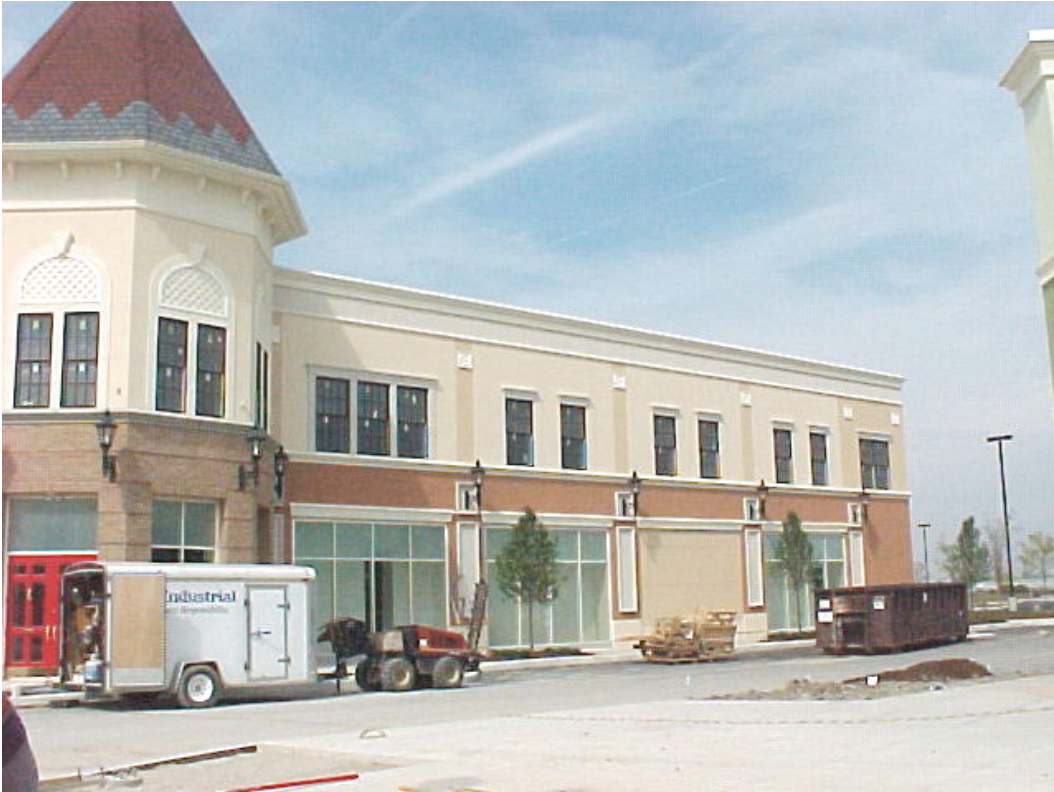
Looking Northwest Bldg #200
