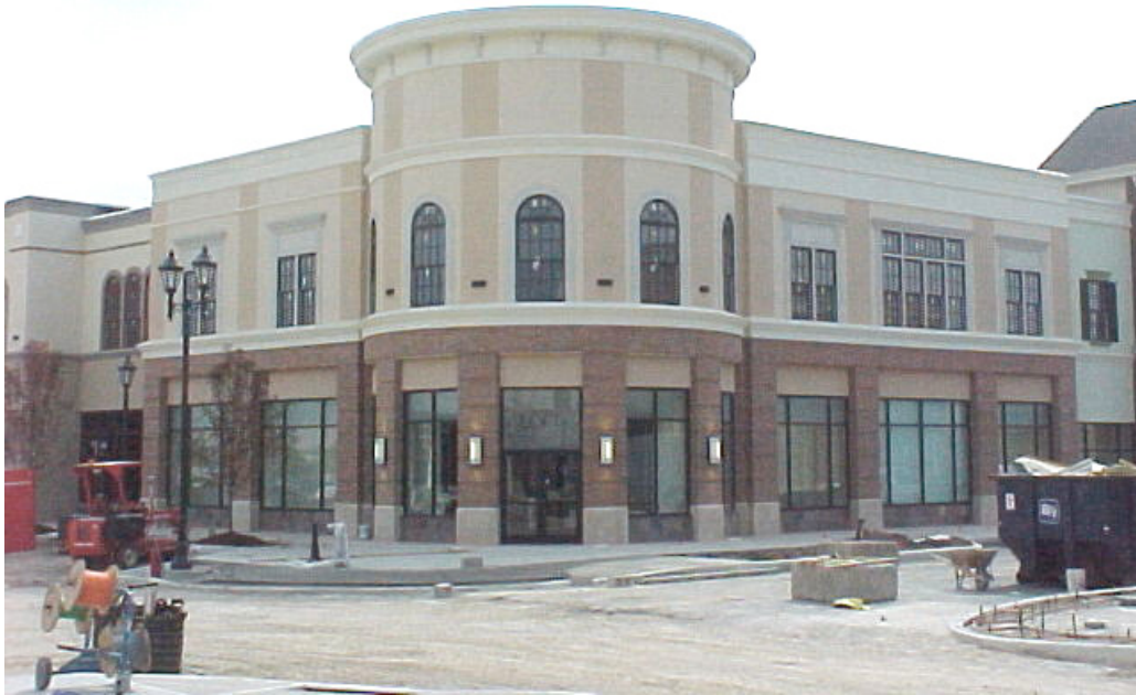
Looking Southeast Bldg #1100 – Ann Taylor Loft
