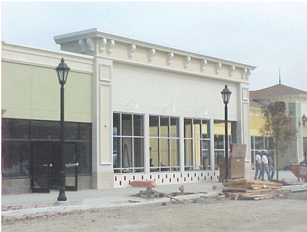
Looking Northeast Bldg #500 - Johnny Rockets
