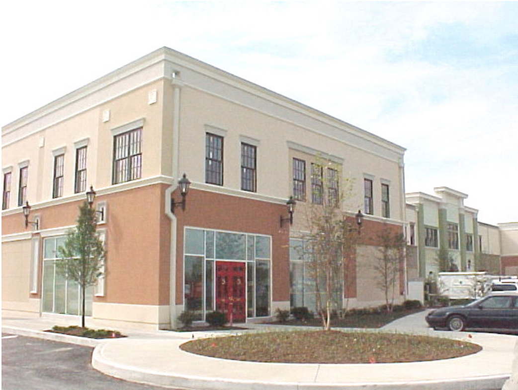
Looking Southwest Bldg #200 / rear of Talbots
