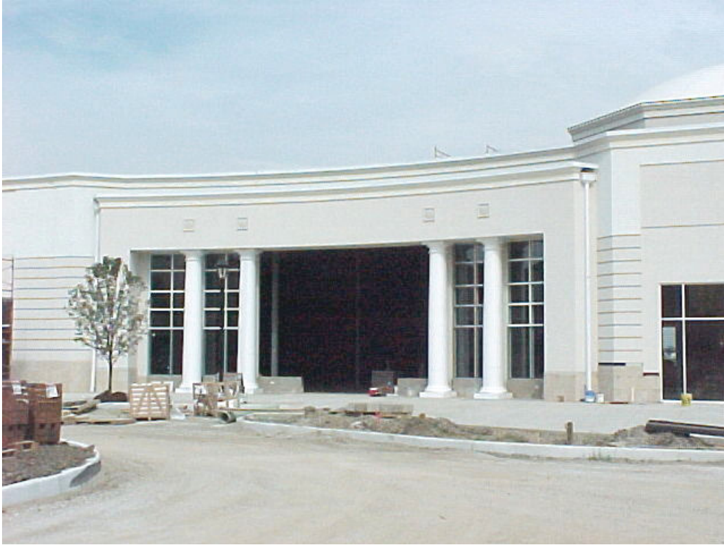
Looking North Bldg #100
