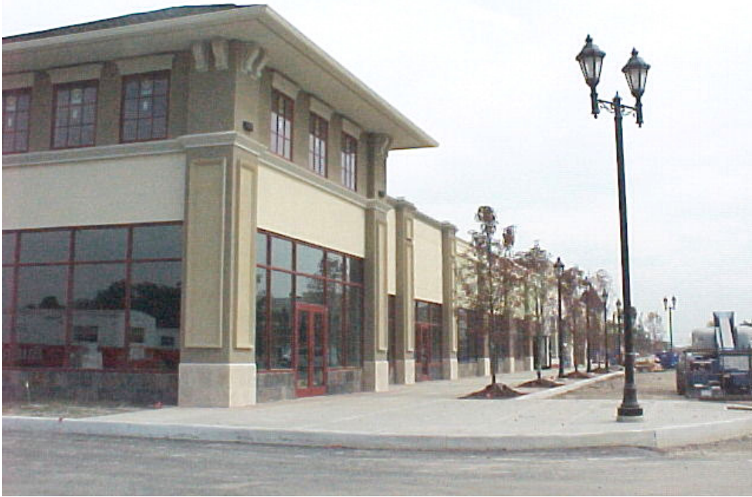
Looking Northeast Bldg #500
