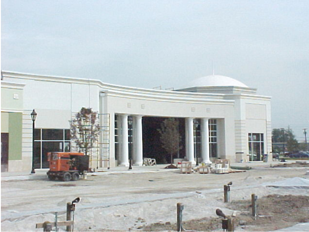
Looking Northeast Bldg #100
