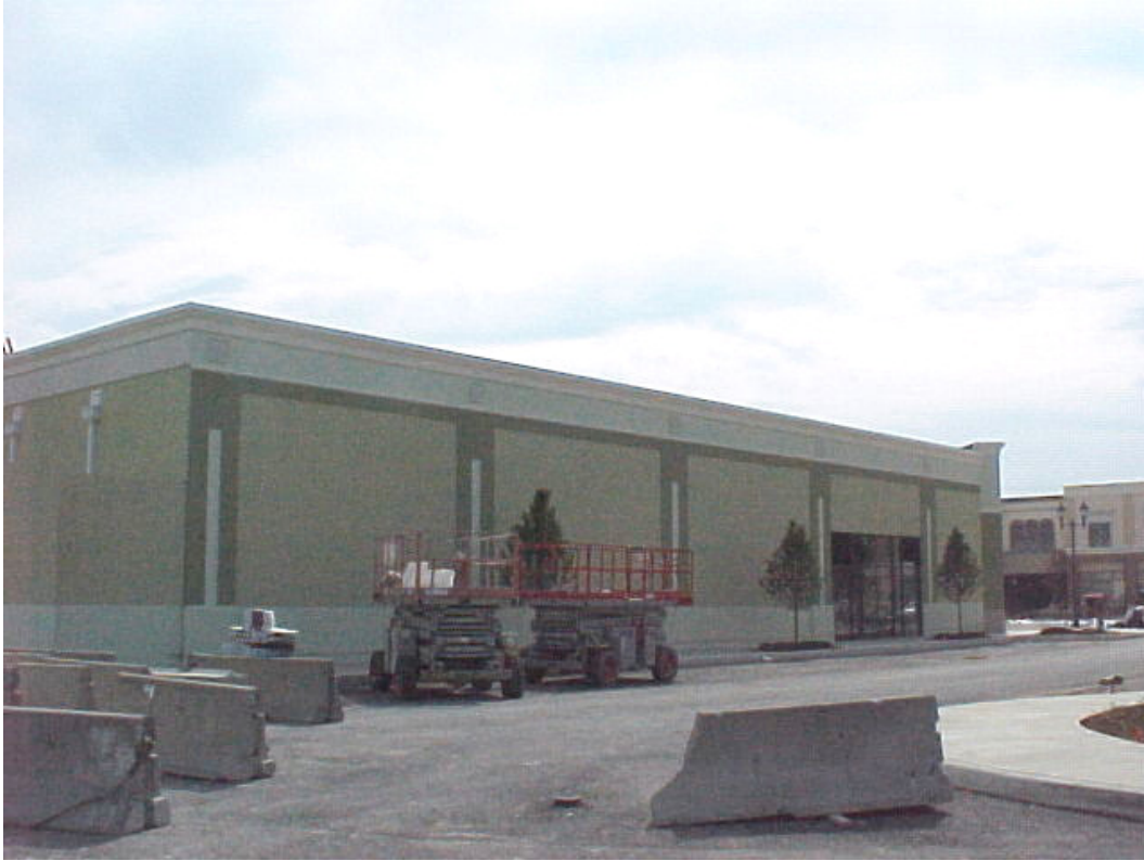
Looking Southeast Bldg #100
