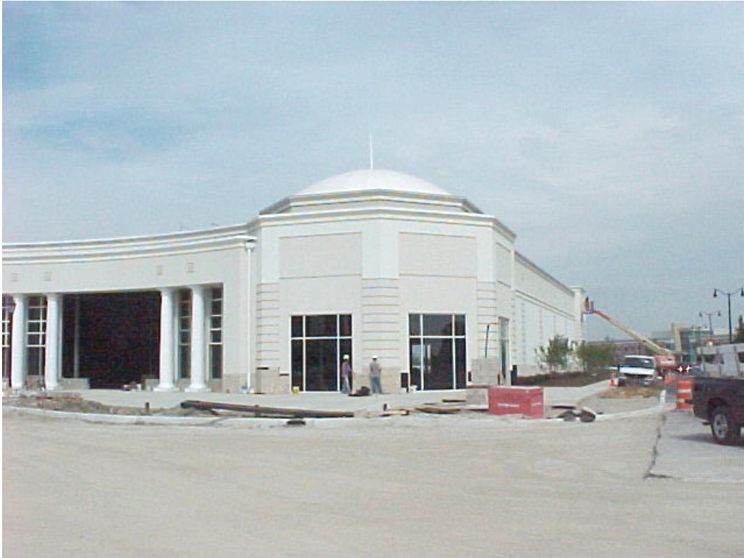
Looking North Bldg #100
