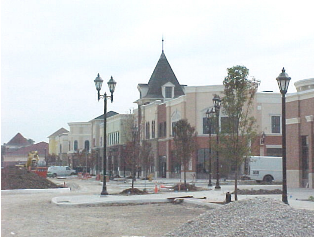
Looking Southeast Bldg #800
