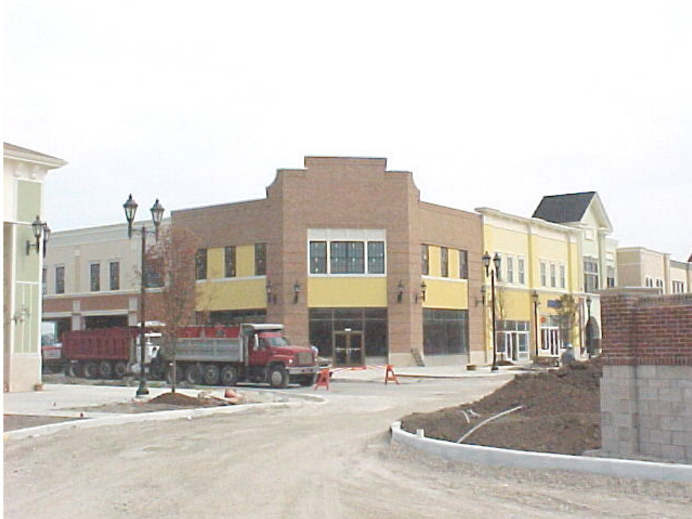
Looking Northeast Bldg #200
